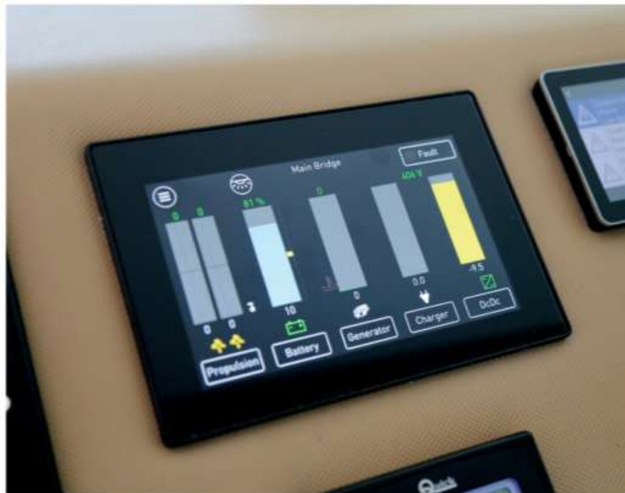
The Silent 60’s engine room is highly accessible and beautifully designed—as is its energy consumption interface.
